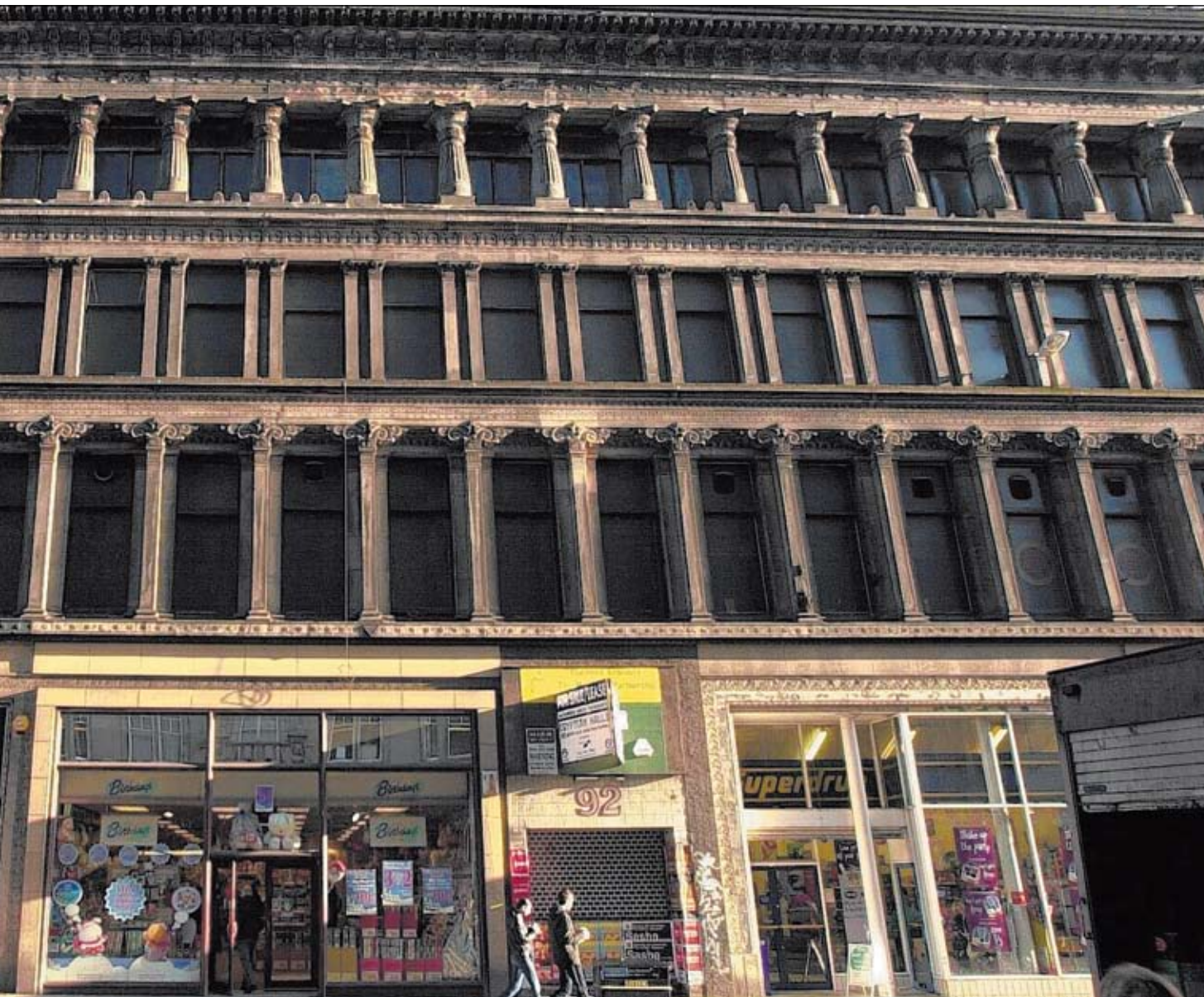
■ The plan would create a hotel from the building which has lain derelict for almost 30 years
